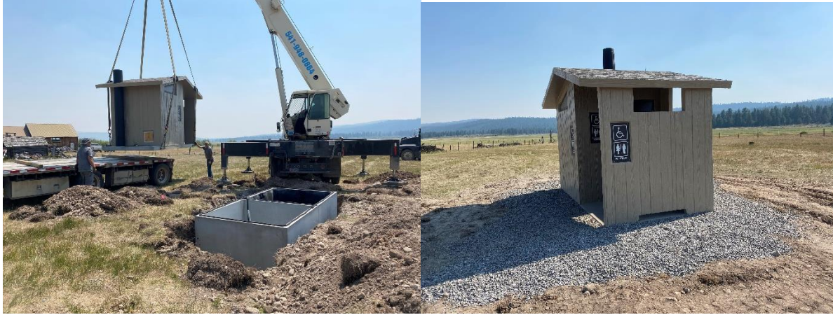
Figure 3.2.1. Vault toilet installed at Logan Valley on July 13 th , 2021.
