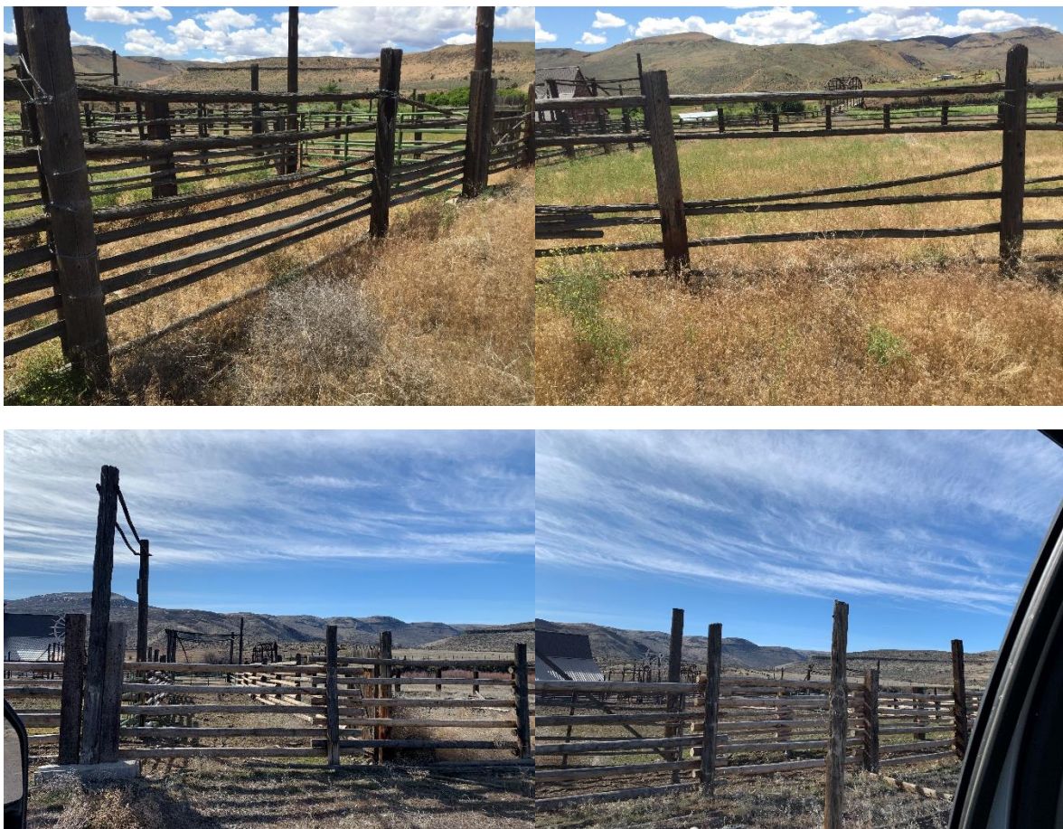
Figure 3.2.1. Corral photos in June 2020 (top) and February 2022 (bottom). We have replaced dilapidated crossbars with new lodgepole pine crossbars.
