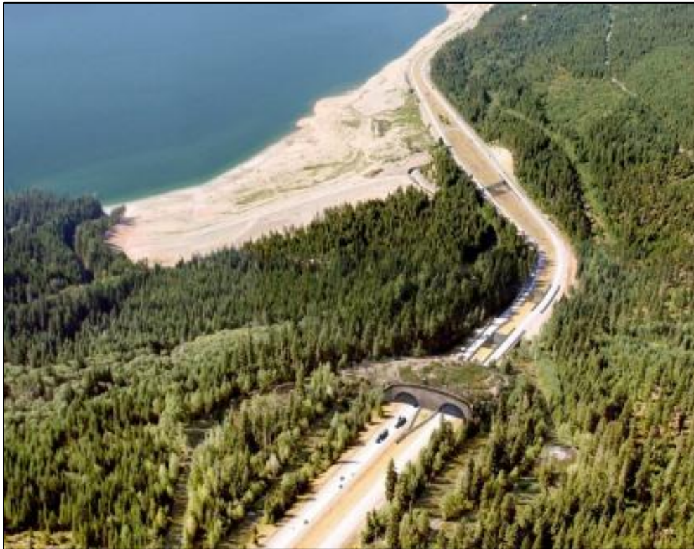
Figure 12. Wildlife Underpass at an Aquatic Culvert Crossing Facilitating Both Fish and Wildlife Movement
