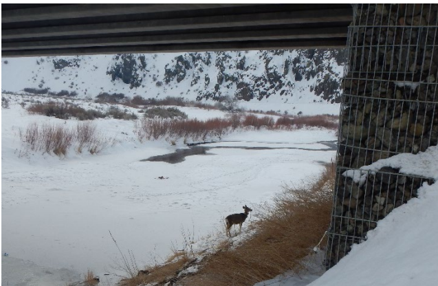
Figure 7. Mule deer using bank under bridge 19915 as passage
