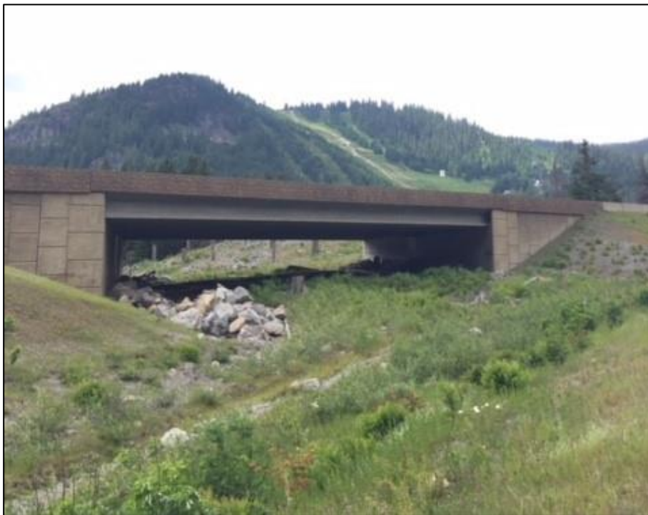
Figure 11. Examples of a Wildlife Underpass Facilitating Wildlife Movement And Habitat Connectivity under Interstate 90 in Washington State
