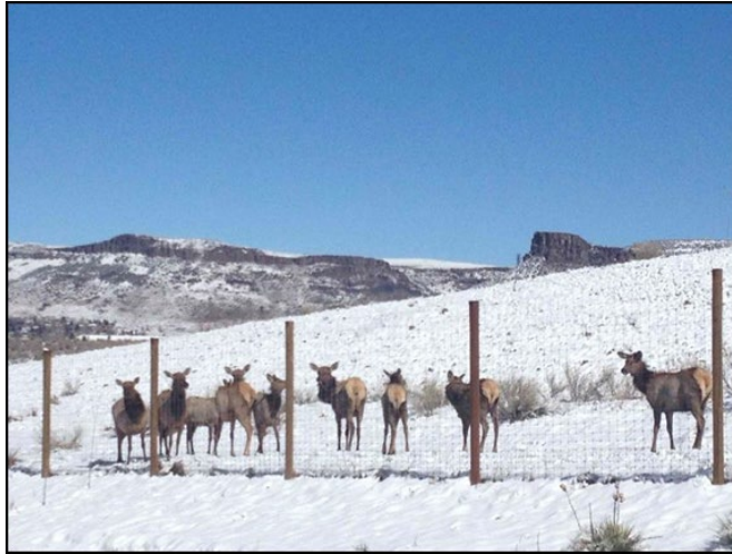
Figure 3. Eight-foot high large mammal exclusion fencing, CO.© J. Kintsch
