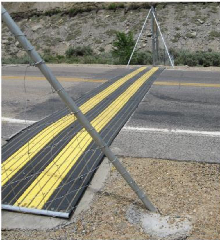
Figure 19. CrossTek™ Electric Wildlife Mat™ at a Highway Crossing in Utah
