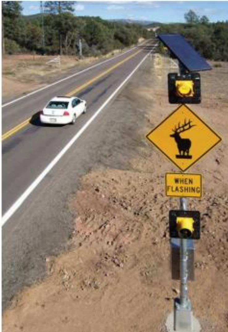
Figure 24. Photo of a CrossTek™ Animal Detection System At-Grade Crosswalk
