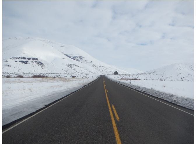
Figure 6. Typical road profile on Highway 20
