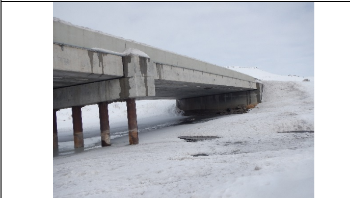
Photo 5. 19910: Outlet, east-side. During high flow no pathway is available.
