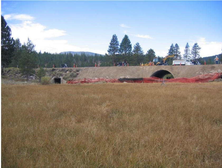
Viewing the old structure adjacent to the newly constructed Kyburz Flat underpass. Photo Credit: US Forest Service
