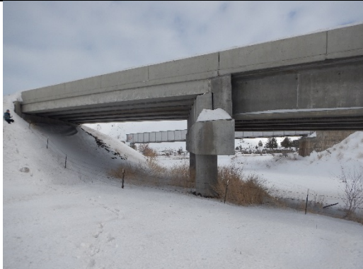
Photo 1. 19908: Eastern edge of inlet side. Note large dry pathway interrupted by wire strand fence.
