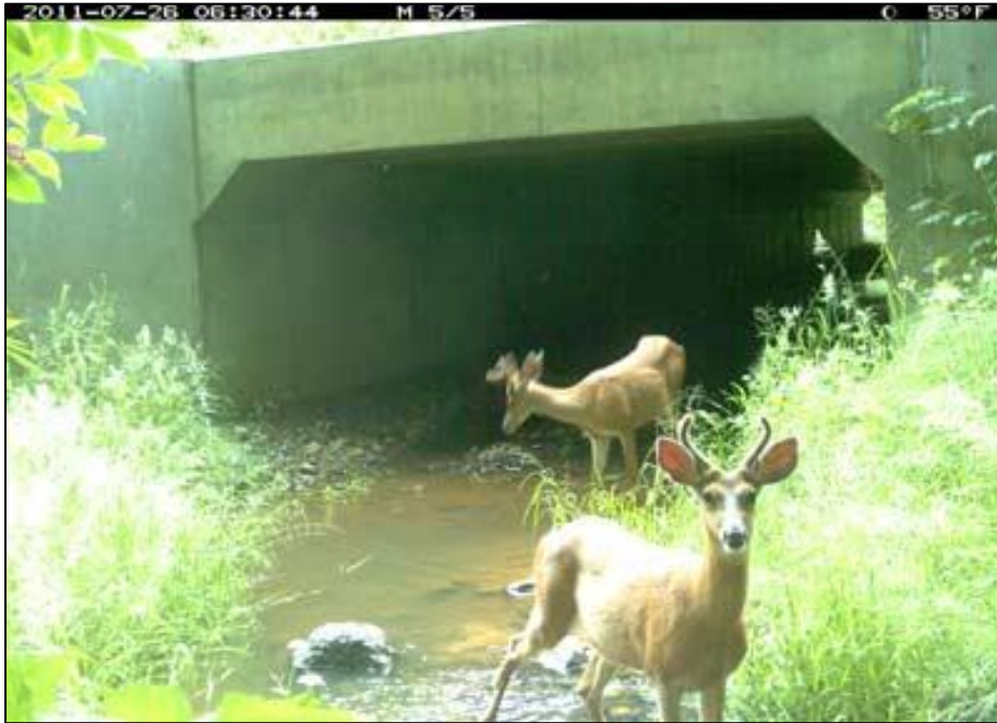
Figure 12. Wildlife Underpass at an Aquatic Culvert Crossing Facilitating Both Fish and Wildlife Movement
