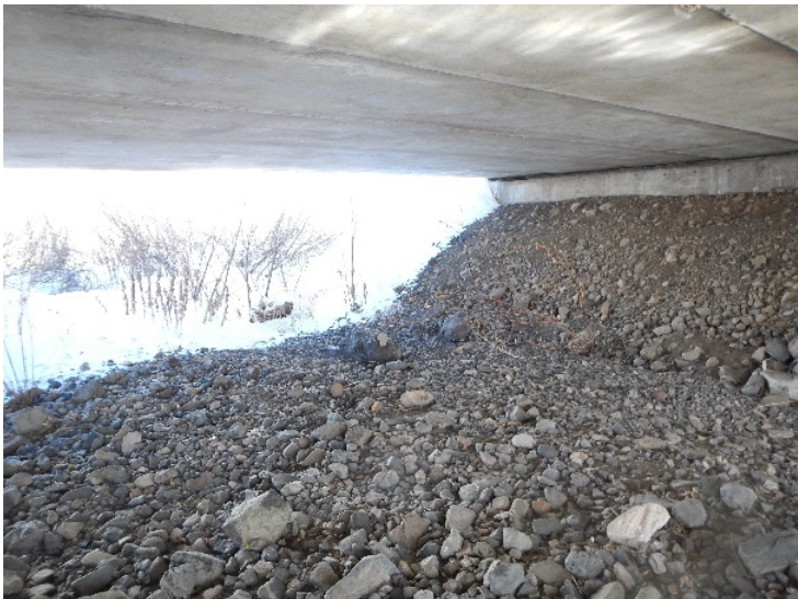
Figure 1. Extensive stream bed material under bridge
