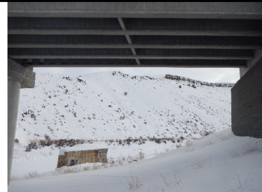
Photo 4. 19909: Outlet side. Dry, mostly-level pathway on west side.
