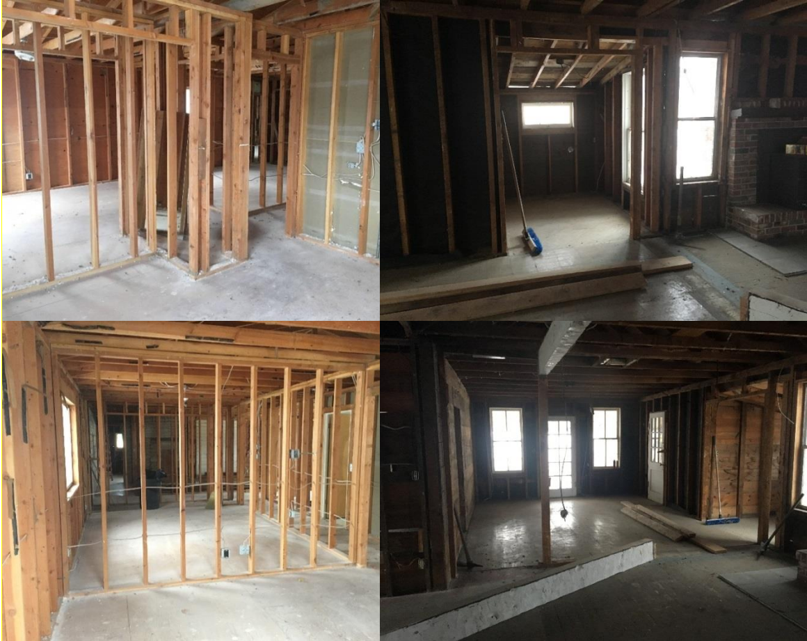
Figure 3.3.1. Bunkhouse renovations in progress 2018.
