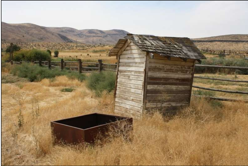
East and north sides, looking southwest
