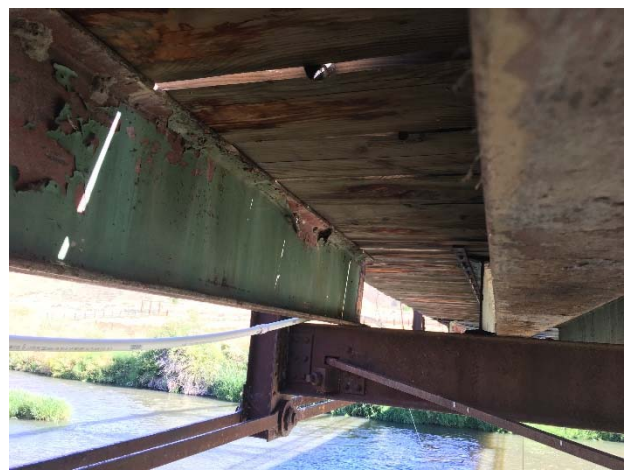
Photo 10. Bridge Pin/Eyebare Connection
