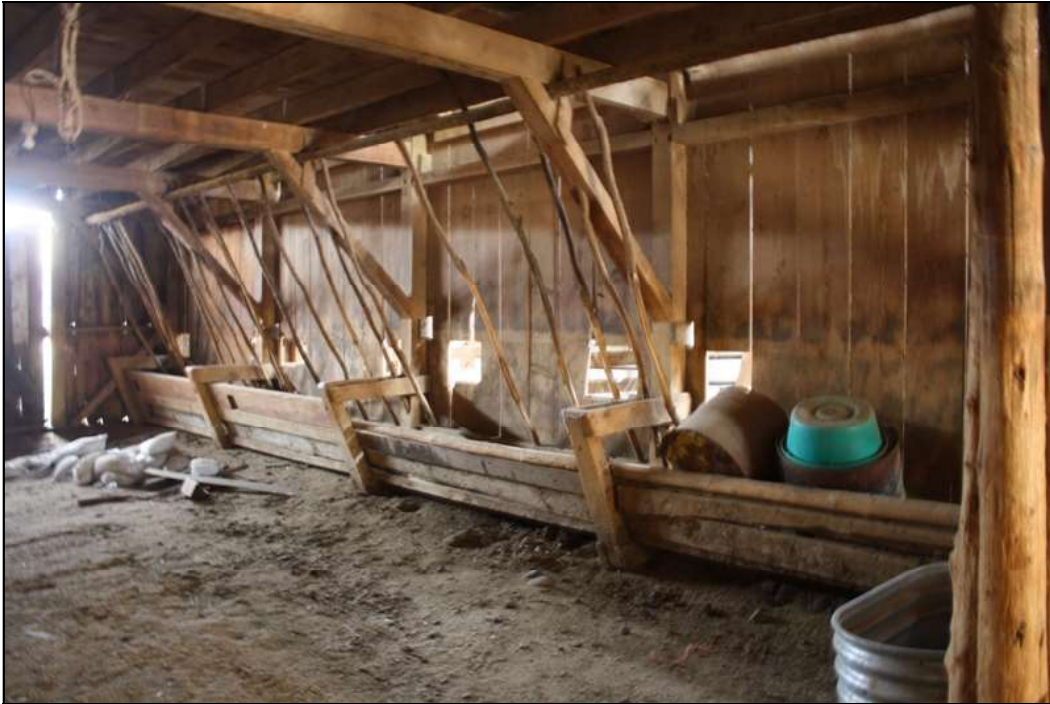
Mangers, central aisle, north side, west end, looking northwest
