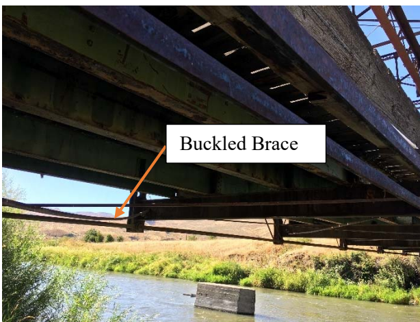
Photo 9. Bridge Deck Bracing
