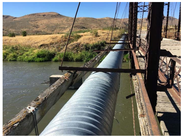
Photo 8. Irrigation Pipe Suspended From Bridge
