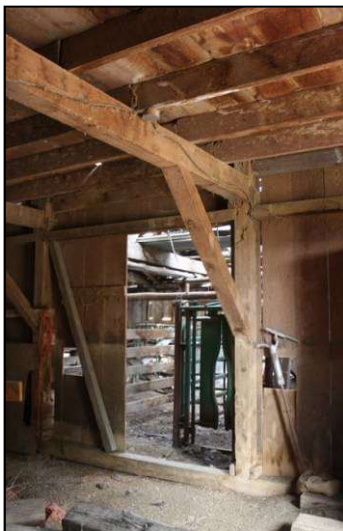
Interior bents, looking northwest
