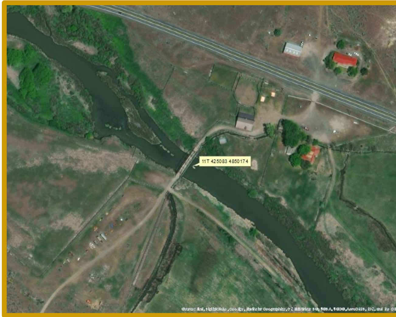
Figure 6. Bridge Location at MRWMS.
