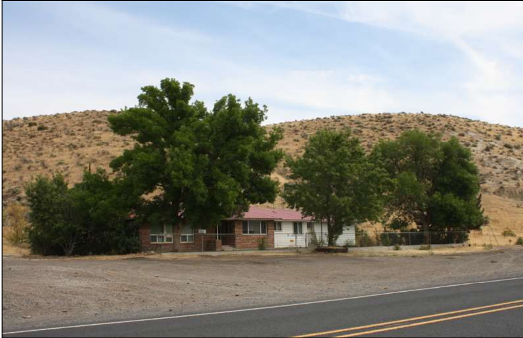
Front (south) façade, looking northeast
