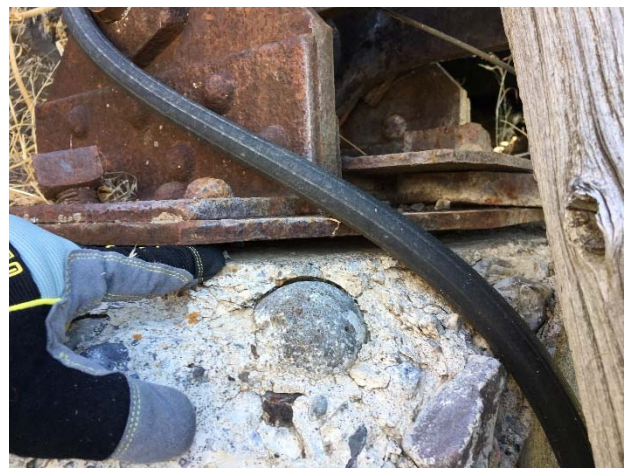
Photo 18. Rotated Bearing Plate (NW Corner)
