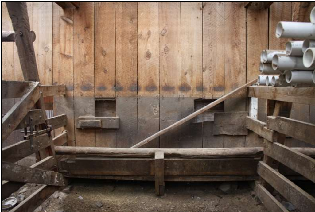
North aisle, stall with manger, looking south
