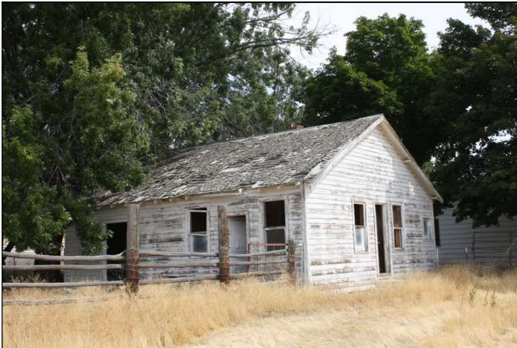
Bunkhouse, west and south facades
