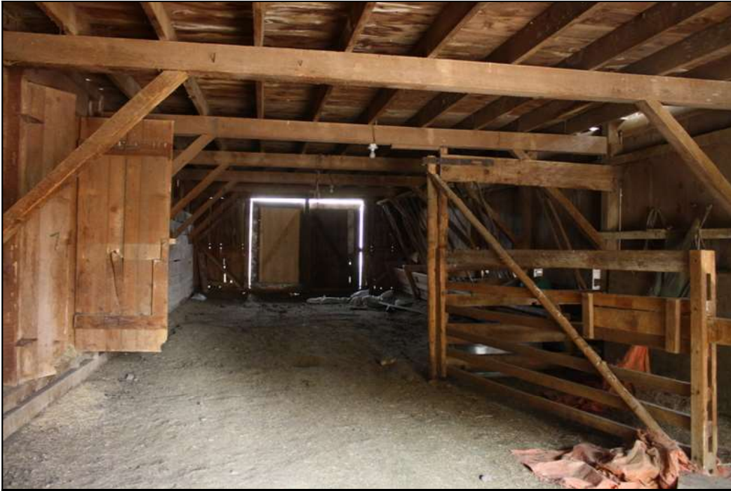
Central aisle, facing west, showing timber bents
