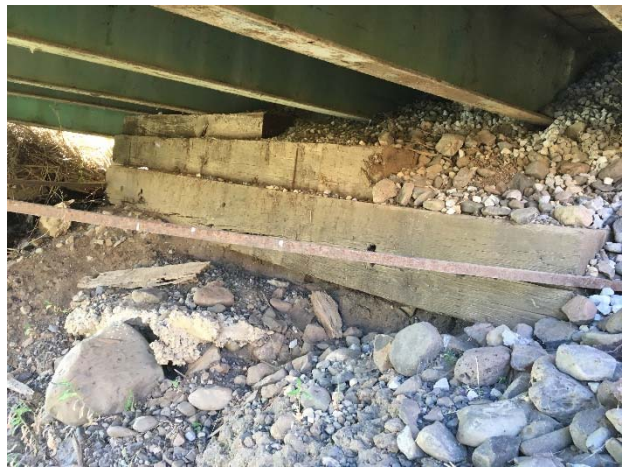
Photo 14. South Abutment Stringer Supports
