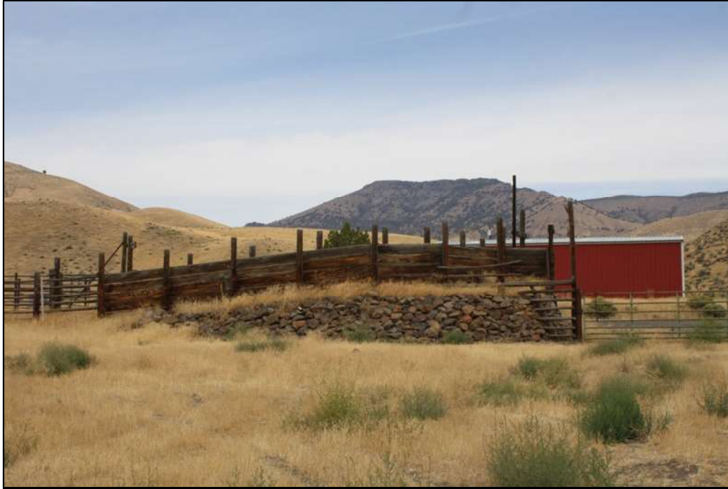
Main loading chute, looking north
