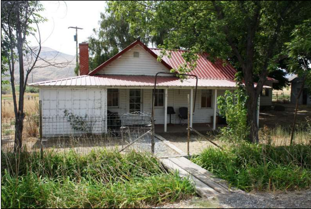
North (front) façade, east end, looking south
