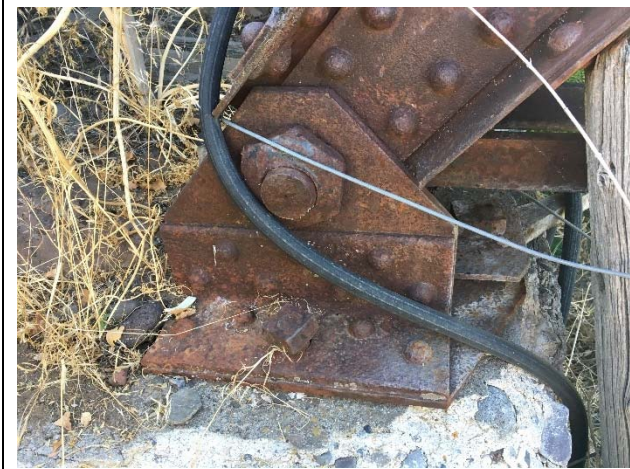
Photo 17. Typical Pin Bearing (NW Corner)
