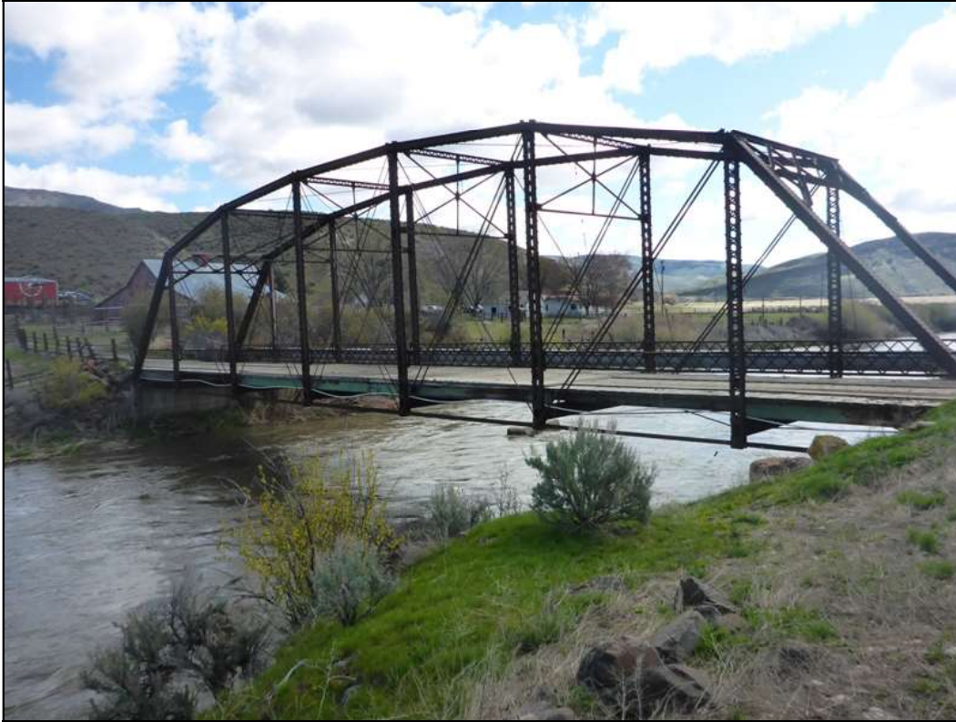
East side of bridge, looking west
