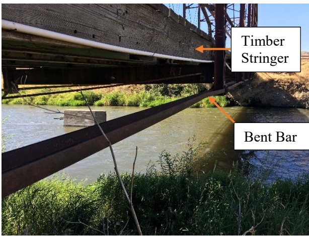
Photo 7. Bridge Bottom Chord
