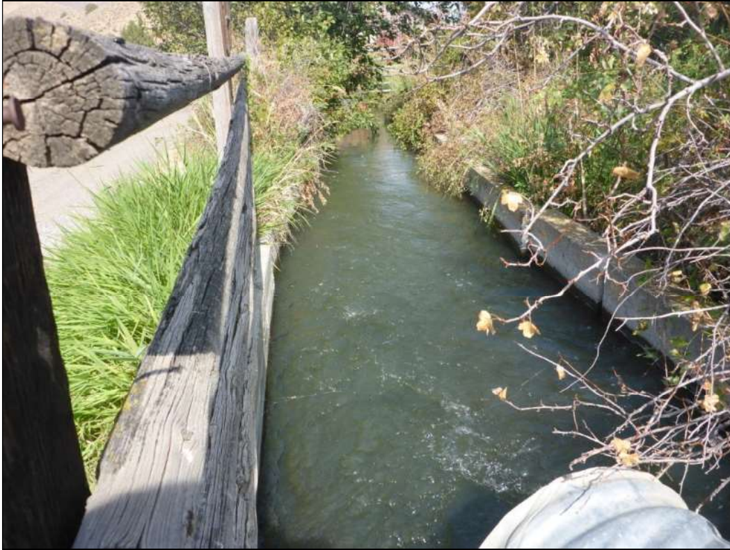
Irrigation ditch as it emerges from pipe on north side of bridge, looking north
