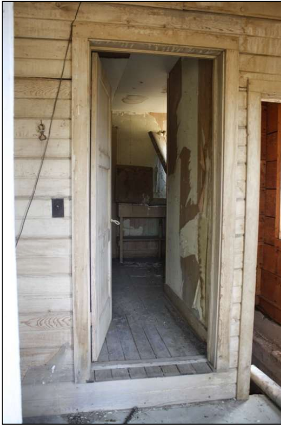
Main entry from enclosed porch, looking east
