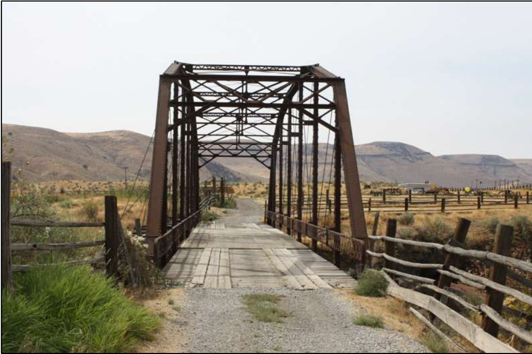
North approach to bridge, looking south
