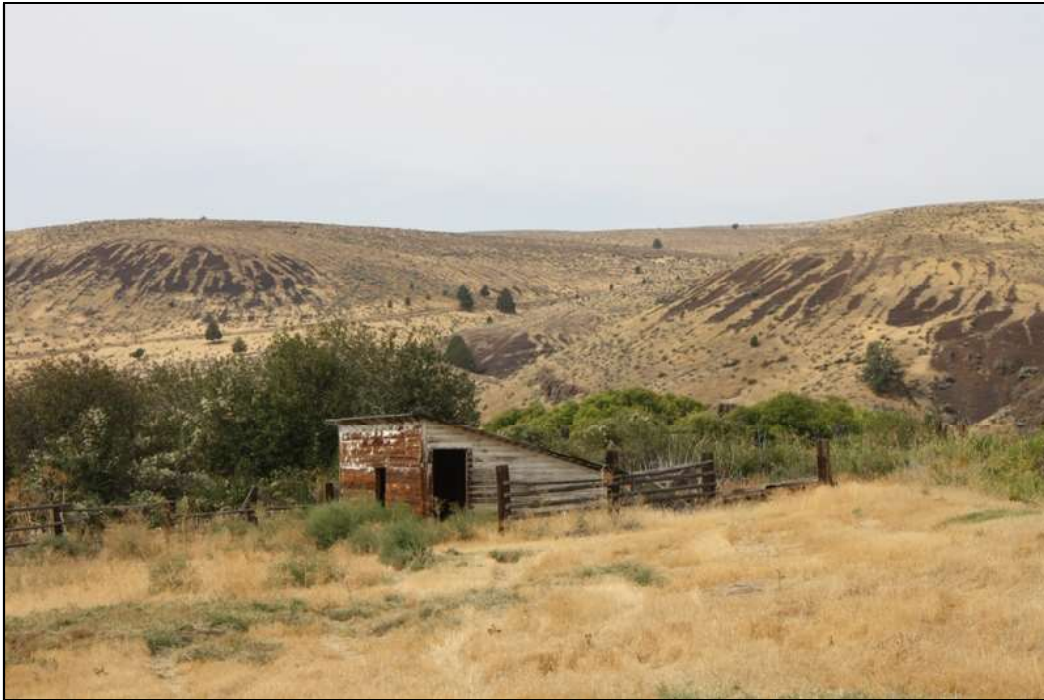
South and east (entry) facades, looking northwest
