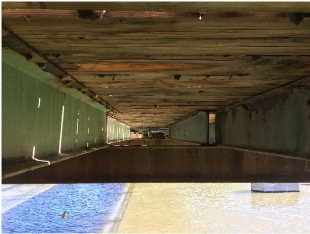
Photo 11. Bridge Floor Beam and Stringers
