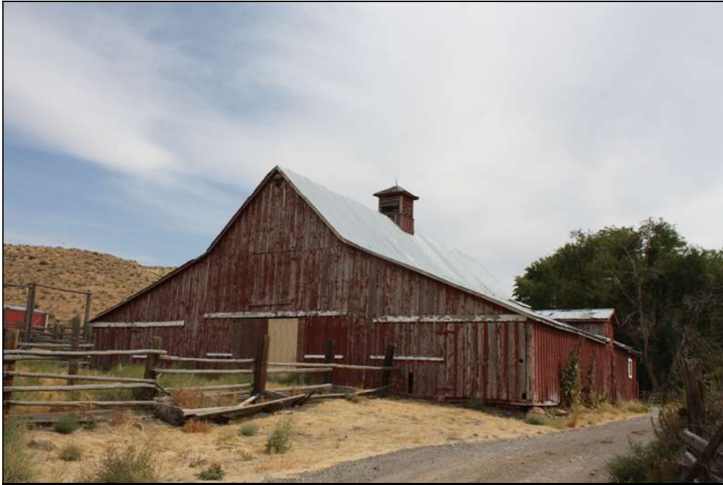
West (rear) and south side facades, looking east
