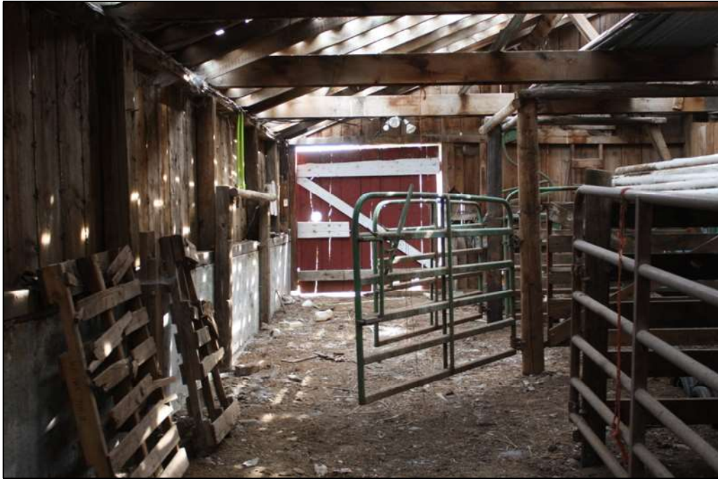
North aisle, looking east, metal gates for stalls to the right
