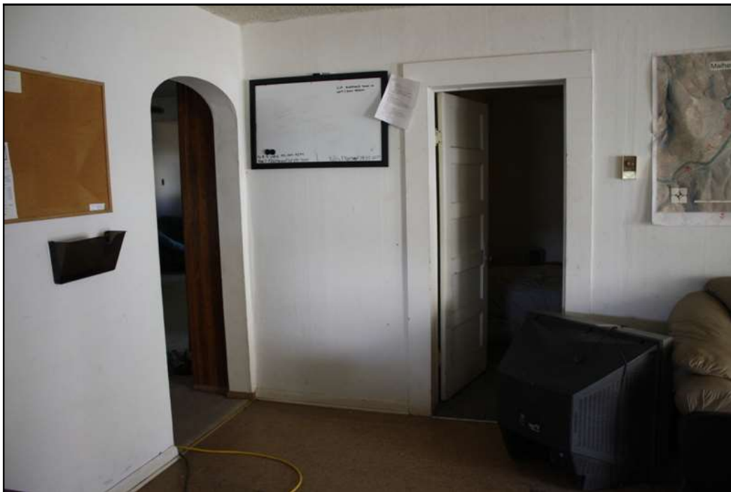
Main entry room, looking south
