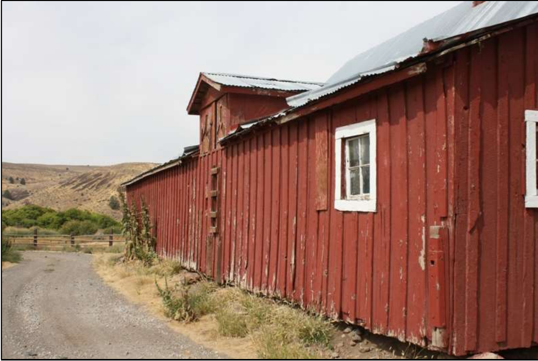
South side façade, looking west
